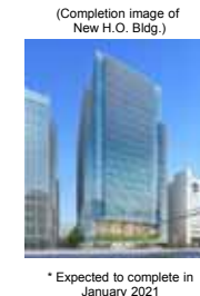
* Expected to complete in January 2021
