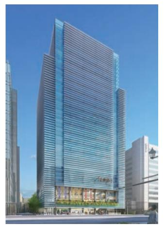
We plan to introduce the state-of-the-art environmental technologies for new Head Office building to be completed in January 2021. We aim for creating an environmentally friendly office building by applying a natural ventilation system where a building itself takes in wind by using natural energy, terrestrial heat that keeps the building cool in summer and warm in winter, power-saving LED lights, and rainwater harvesting that saves water resources.
